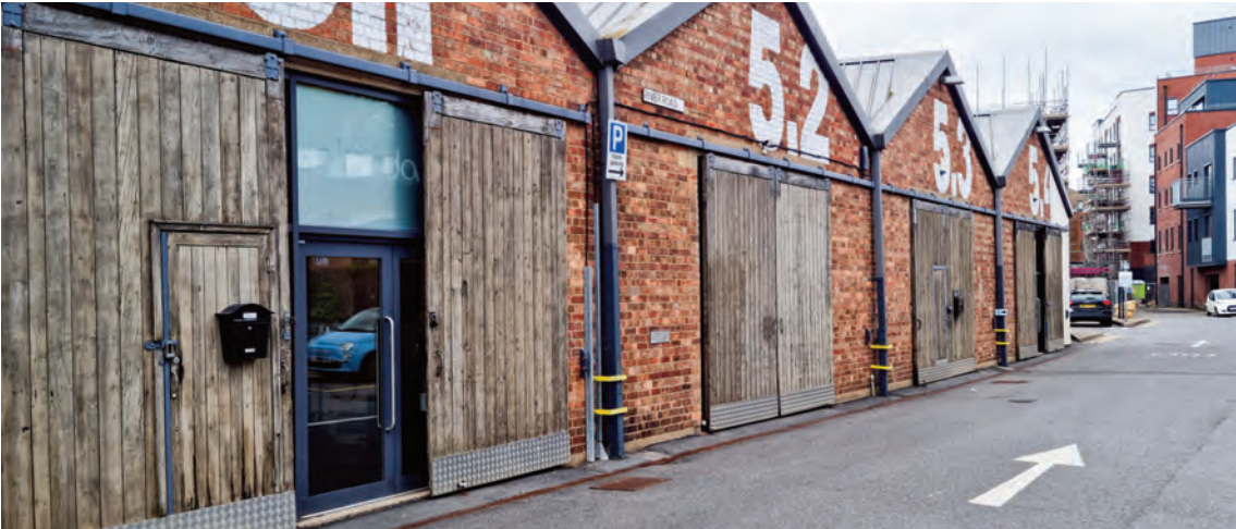
REFURBISHED INDUSTRIAL UNITS (BRISTOL)
