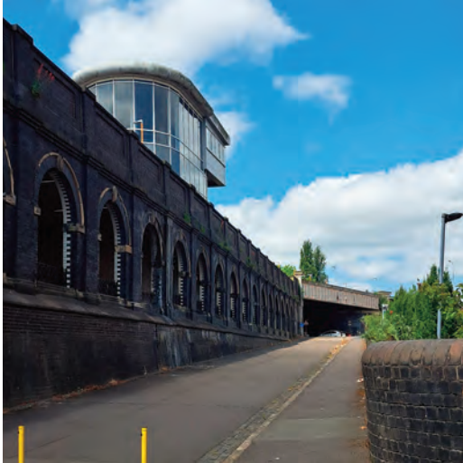
▲ EASTERN SIDE OF WOLVERHAMPTON RAILWAY STATION
