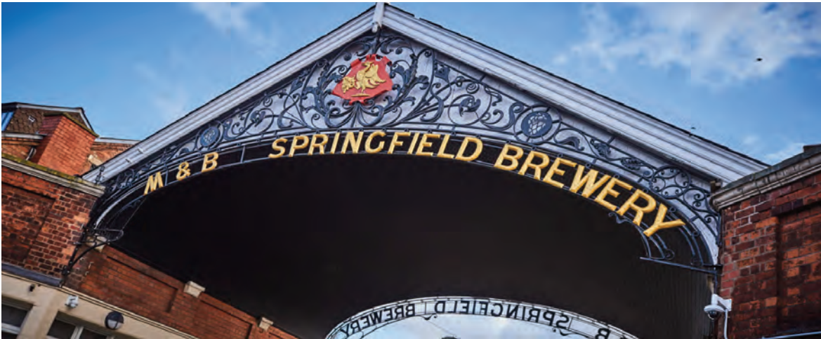
▲ FORMER SPRINGFIELD BREWERY GATE ENTRANCE, PROVIDING ENTRY TO SPRINGFIELD CAMPUS AND THOMAS TELFORD UTC ON CAMBRIDGE STREET
