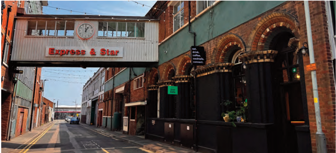
▲ FORMER EXPRESS & STAR NOW WITH CAFE, BAR, RESIDENTIAL AND INDEPENDENT BUSINESS SPACE
