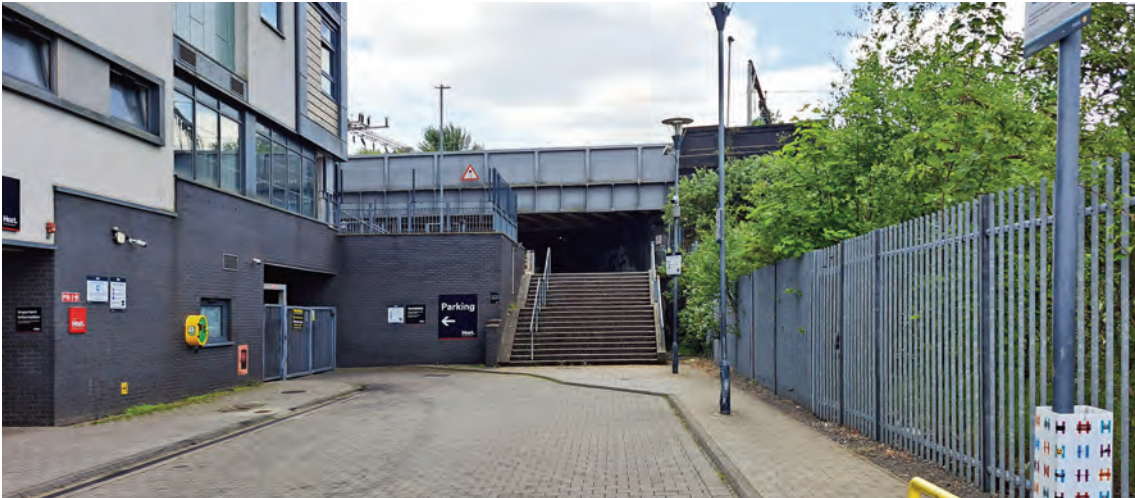
▲ ACCESS IMPROVEMENTS TO LITTLE’S LANE WITH STEP-FREE ACCESS
