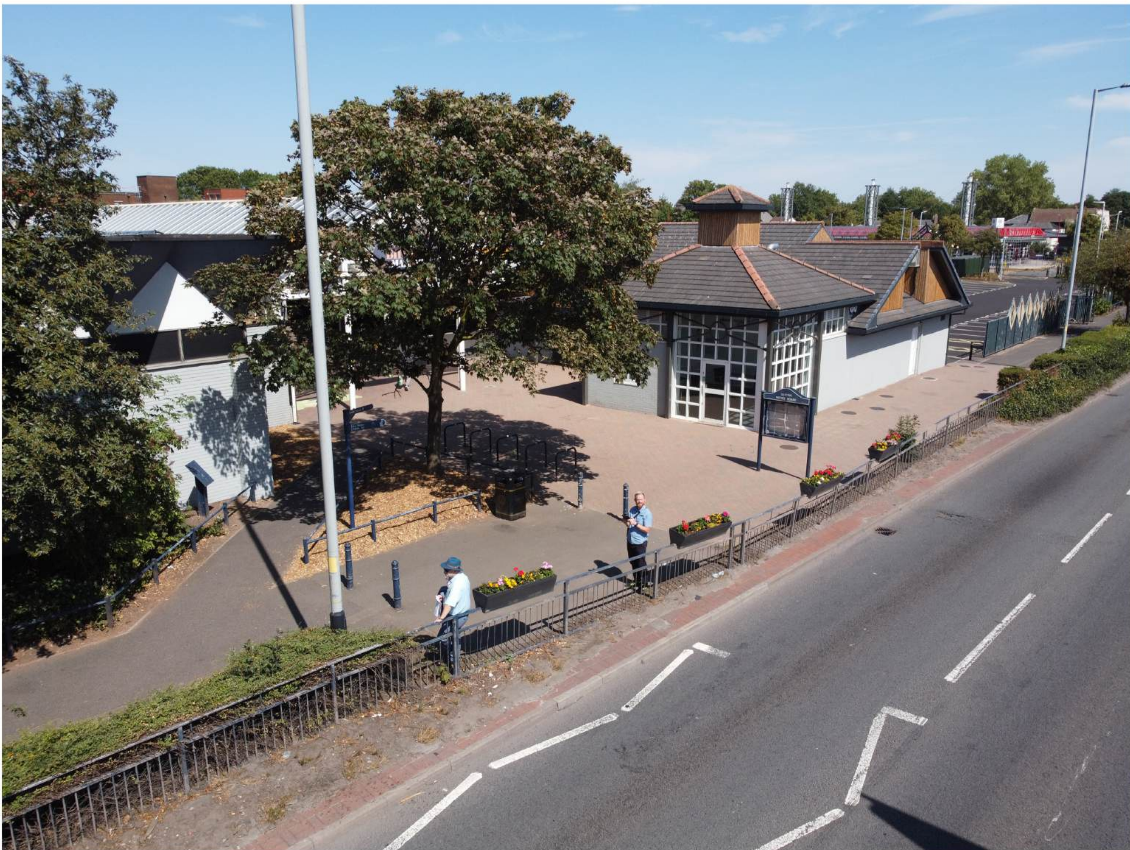
(View from outdoor market entrance before improvements)
